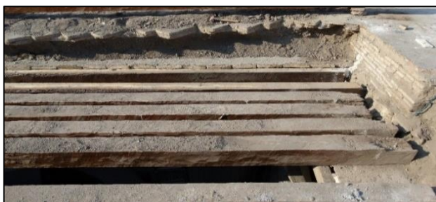
Figure 2. Old beams of the roof framework
